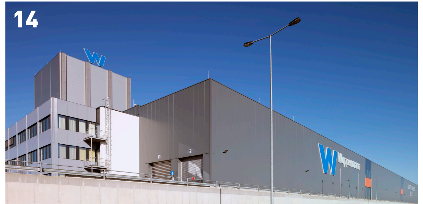
Minimalist design with diverse panel installation gives the architecture a dynamic look. The gray color palette further emphasizes the various activities in the buildings.
