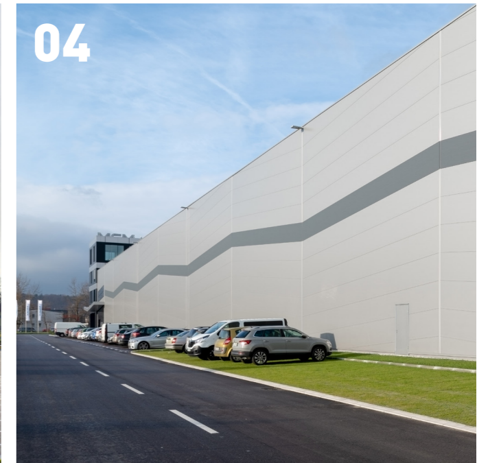
Facade products allowing the installation of openings aligned with the facade surface. Diagonally installed Trimoterm FTV HL panels are up to 14m long.
